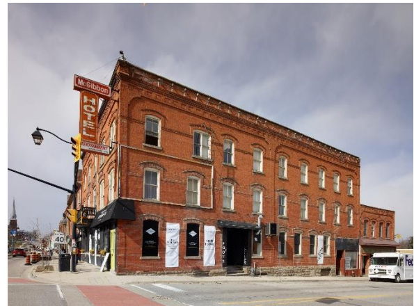
McGibbon Condominium, Georgetown, ON (Photography by Scott Norsworthy)
