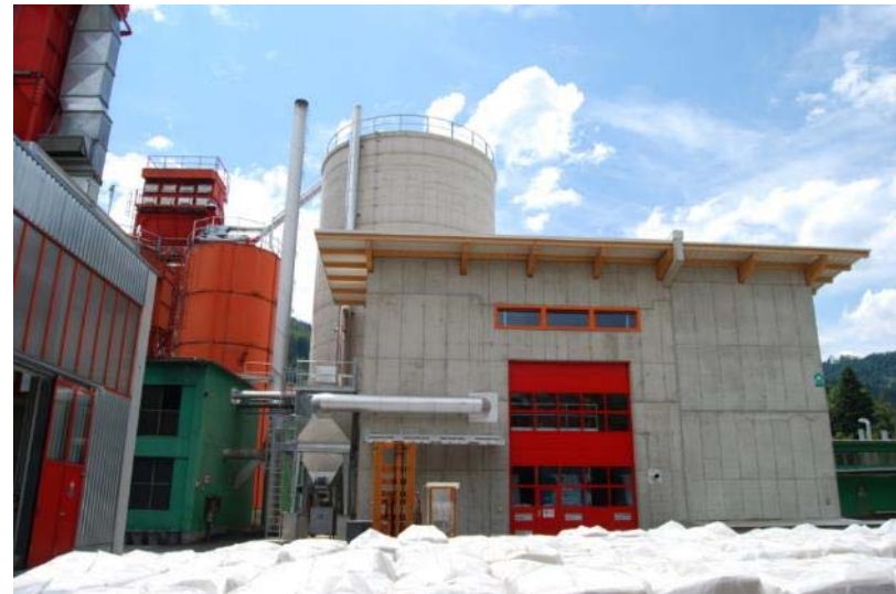
Heating plant - Übelbach
